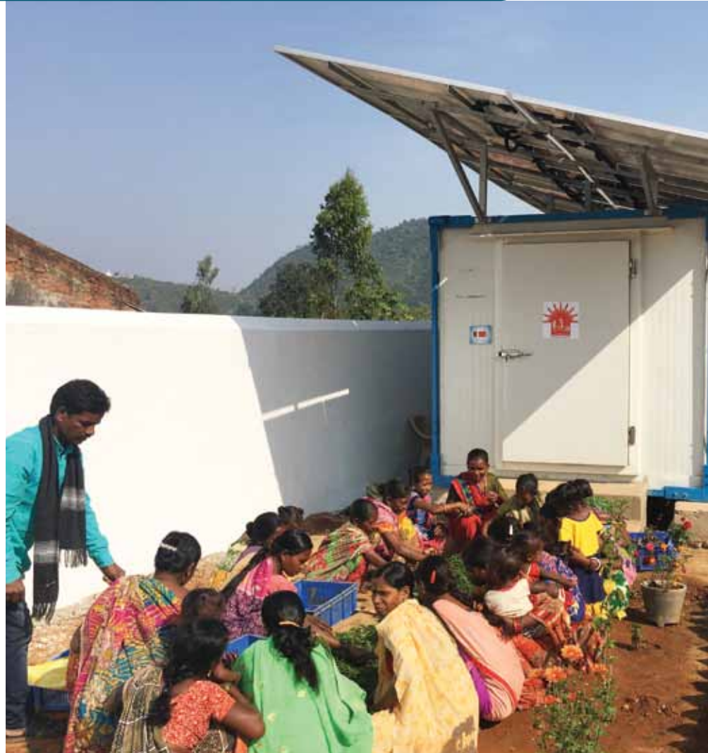
A cold-storage unit based on decentralised renewable energy in an Assam village
